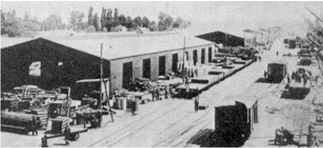
Unloading supplies from ships at a base depot in France, 1918.
